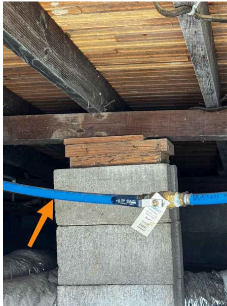
Supply lines not insulated
