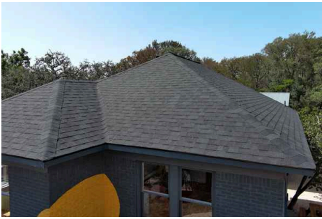
New roof installation
