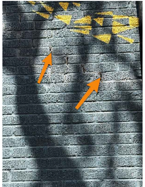
Step fractures still present
