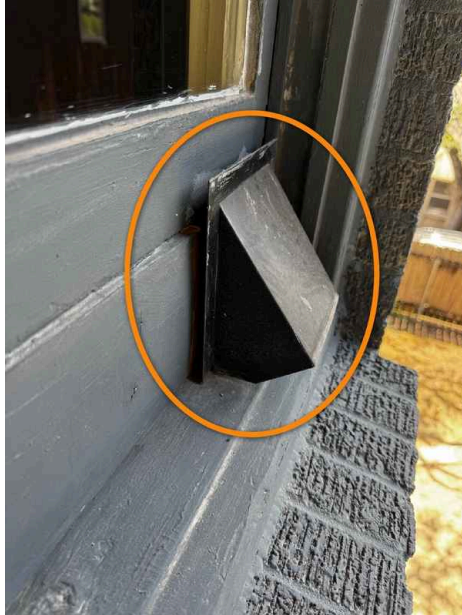
Improper dryer exhaust connection
