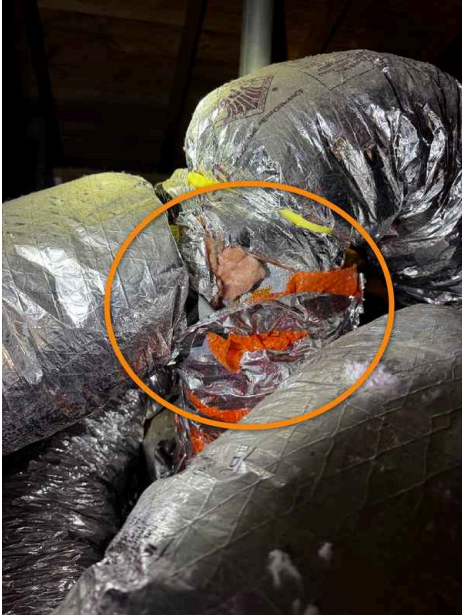
Sweating at HVAC connections
