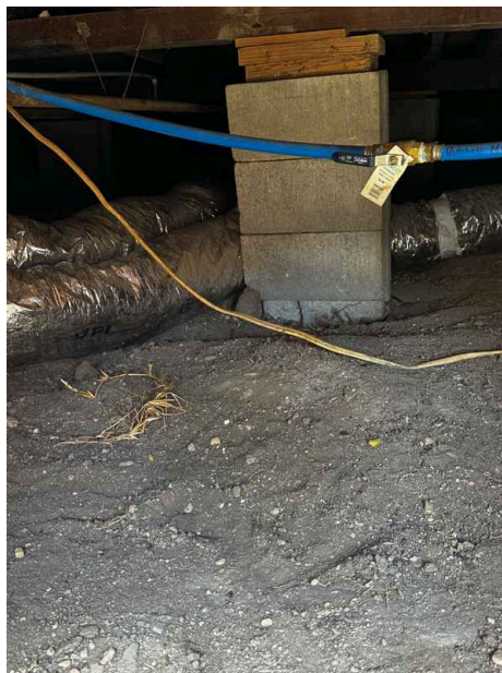
Supply lines not insulated
