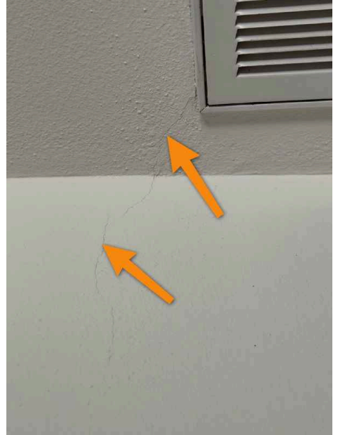
Lateral cracking
